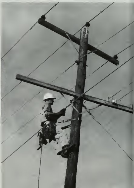
J. T. Burchette, a lineman, works on a joint-use pole, which the telephone company shares with the REA electric cooperative.
